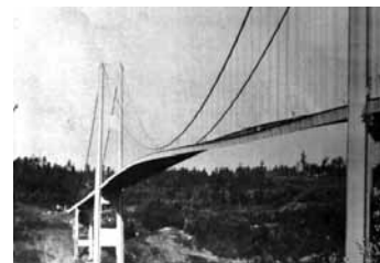
Figure 59: The collapse of the Tacoma Narrows Bridge in 1940 due to wind-induced vibrations.
